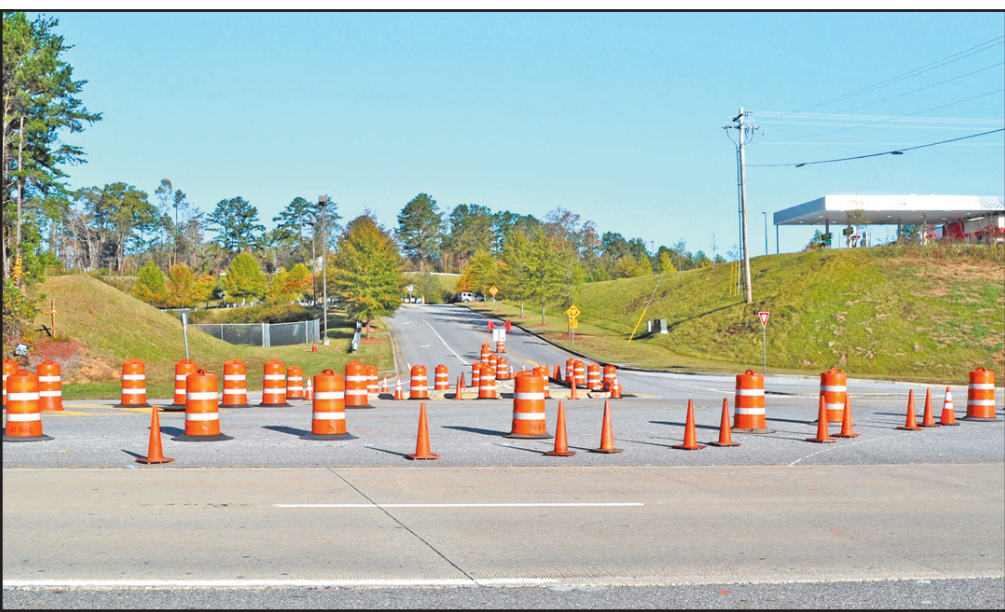
The new exit protocol put in place by the Georgia Department of Transportation will feature traffic upgrades at the Kiutuestia Creek Road and Georgia 515 intersection. Photo/Lowell Nicholson
